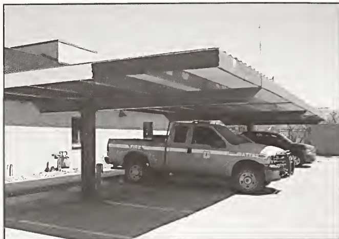
Figure 4—Vehicle exhaust could be drawn into a building's HVAC system if a carport is near the air intake. The air intake for this building is on the roof to prevent vehicle exhaust from being drawn into the Nogales Ranger Station of the Coronado National Forest in the Southwestern Region.
